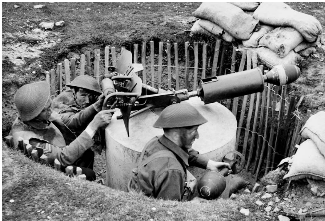
Plate 19. A 29mm Spigot Mortar ('Blacker Bombard'), at No.3 Home Guard Training School, Onibury, Shropshire, May 1943. The reinforced concrete plinth with stainless steel pintle is now the most widespread memorial of the Home Guard. (© IWM)
