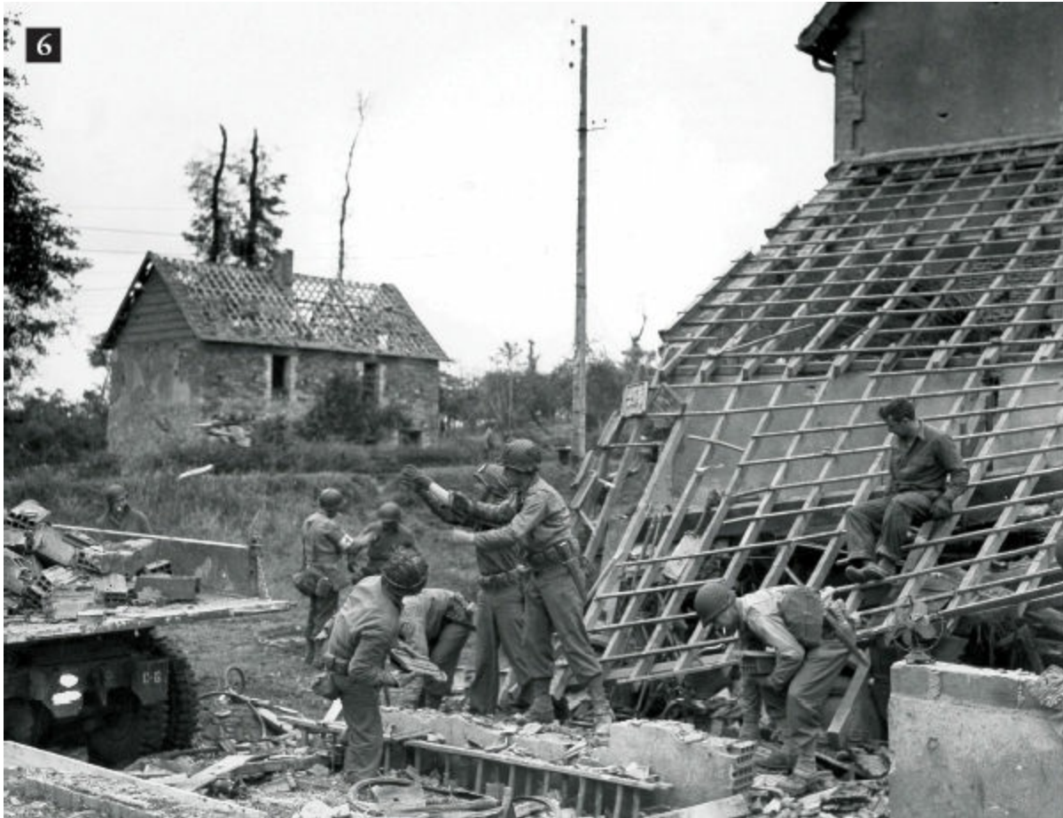
6. Rubble had to be cleared from the roads in order to continue the advance. The soldiers here are clearing a ruined wall and recovering material that could be used to make a new road. The photograph was taken on 11 July, between Saint-Lô and Saint-Fromond. (7171)
