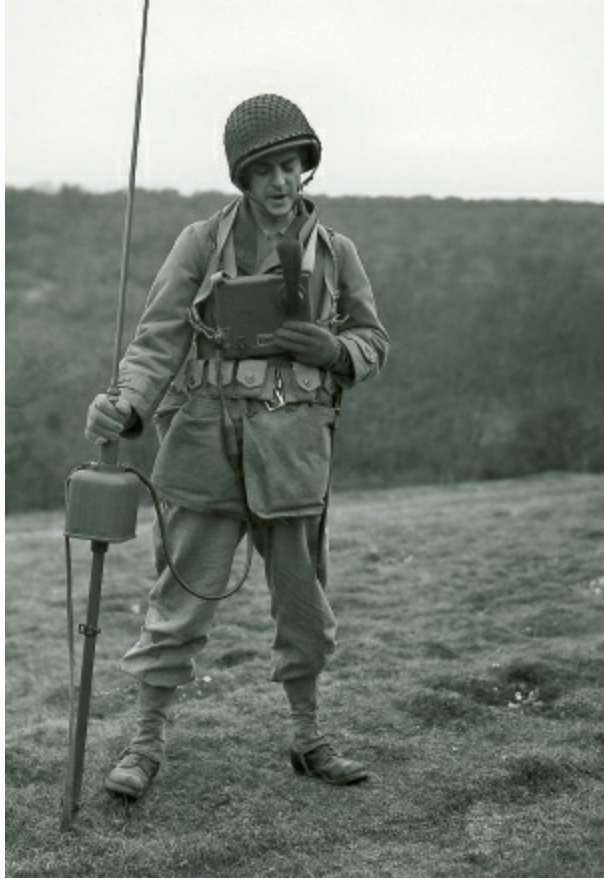
A member of the 121st Engineers Battalion; Ed Lewis, from Steubenville, Ohio. He is carrying a BC-745 radio and holding a 511 model antenna. This photograph was taken on 9 April 1943, near Tidworth. ( DAVA/Coll. Heimdal )
