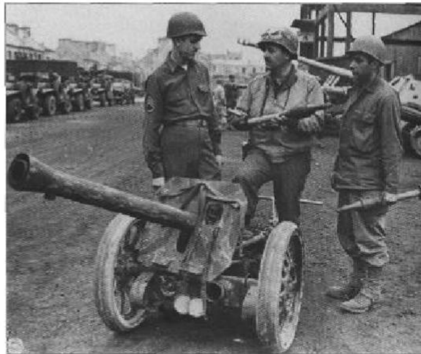
Above: The 8.8cm Raketenwerfer 43, usually called the 'Püppchen', was not a gun but a rocket launcher. It was superseded by the shoulder-held tube rocket launchers,
