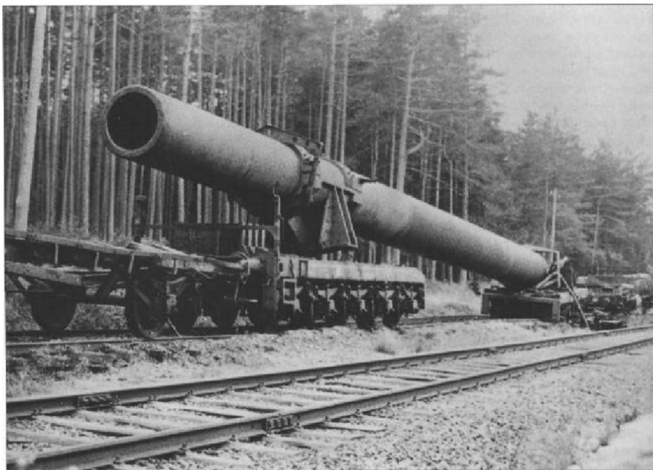
Above: The barrels of very large-calibre guns were transported dismounted. This barrel was captured by Allied forces at the war's end.
