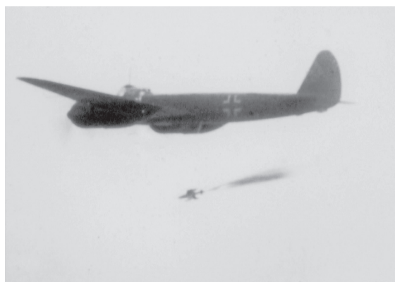
ABOVE Test-firing of the Ruhrstahl X4 V59 from a Ju 88 over the waters of the Baltic during launch trials conducted at Karlshagen. (EN Archive)
