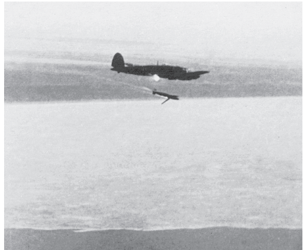
The third prototype Blohm und Voss L 950 torpedo glide-carrier falls away from He 111 DF-0V at 1,000 m during launch tests over the Baltic from Gotenhafen-Hexengrund on 24 April 1942. The rocket motor trigger arm is visible hanging from the lower fuselage of the L 950. This carrier was seen as a progressive development of the L 10 that enabled launching from greater height and longer range, but only seven examples were made before the project was abandoned. (EN Archive)
