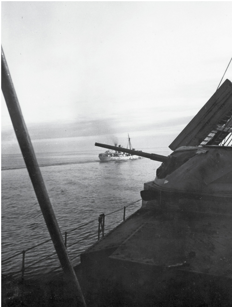
The British armed fishing trawler Ayrshire , as photographed by Ensign Howard E. Carraway from the deck of the Troubadour . In the right foreground is the turret gun of one of the tanks Carraway armed so that it could shoot at planes.
