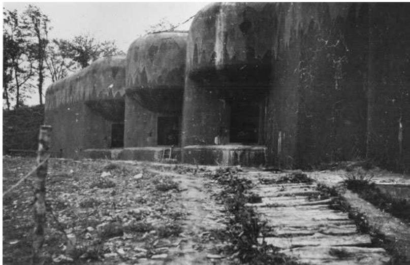
3. An above-ground view of the Maginot Line. Its fortresses were serviced by a highly sophisticated system of underground railways and power stations. As in today's nuclear submarines, the soldiers manning the forts could live like troglodytes without seeing daylight for weeks on end
