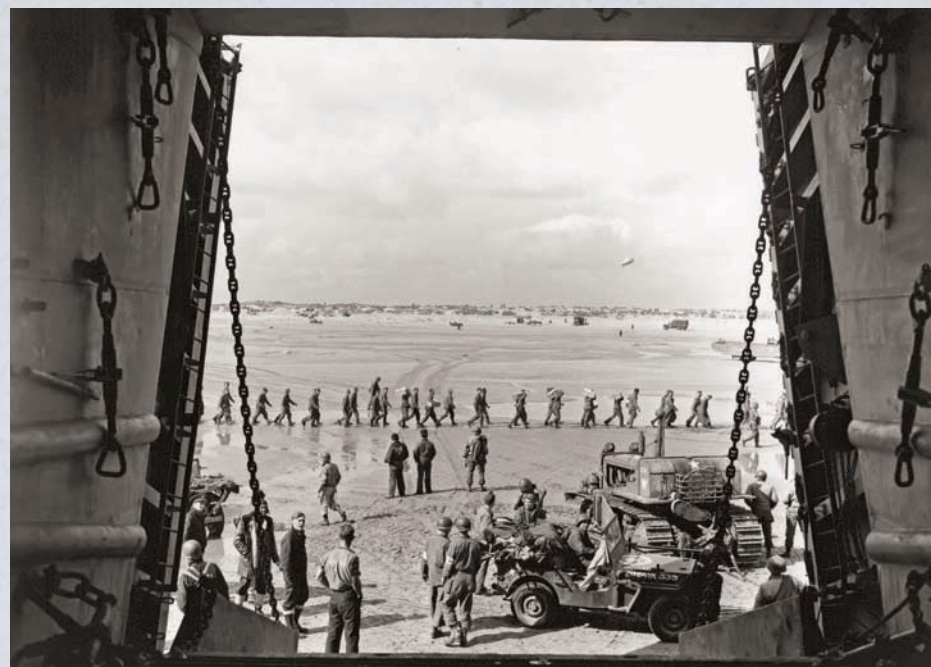
Utah Beach as seen from the tank deck of an LST. At the base of the ramp, two Jeeps have pulled up with casualties for evacuation as a column of German prisoners marches past. Note the U.S. Navy–marked M1 Heavy Tractor/International Harvester TD-18, the DUKW at the center right, and two GMC CCKW 2.5-ton cargo trucks on the beach. U.S. Navy photograph, now in the collections of the US National Archives 80-G-252779
