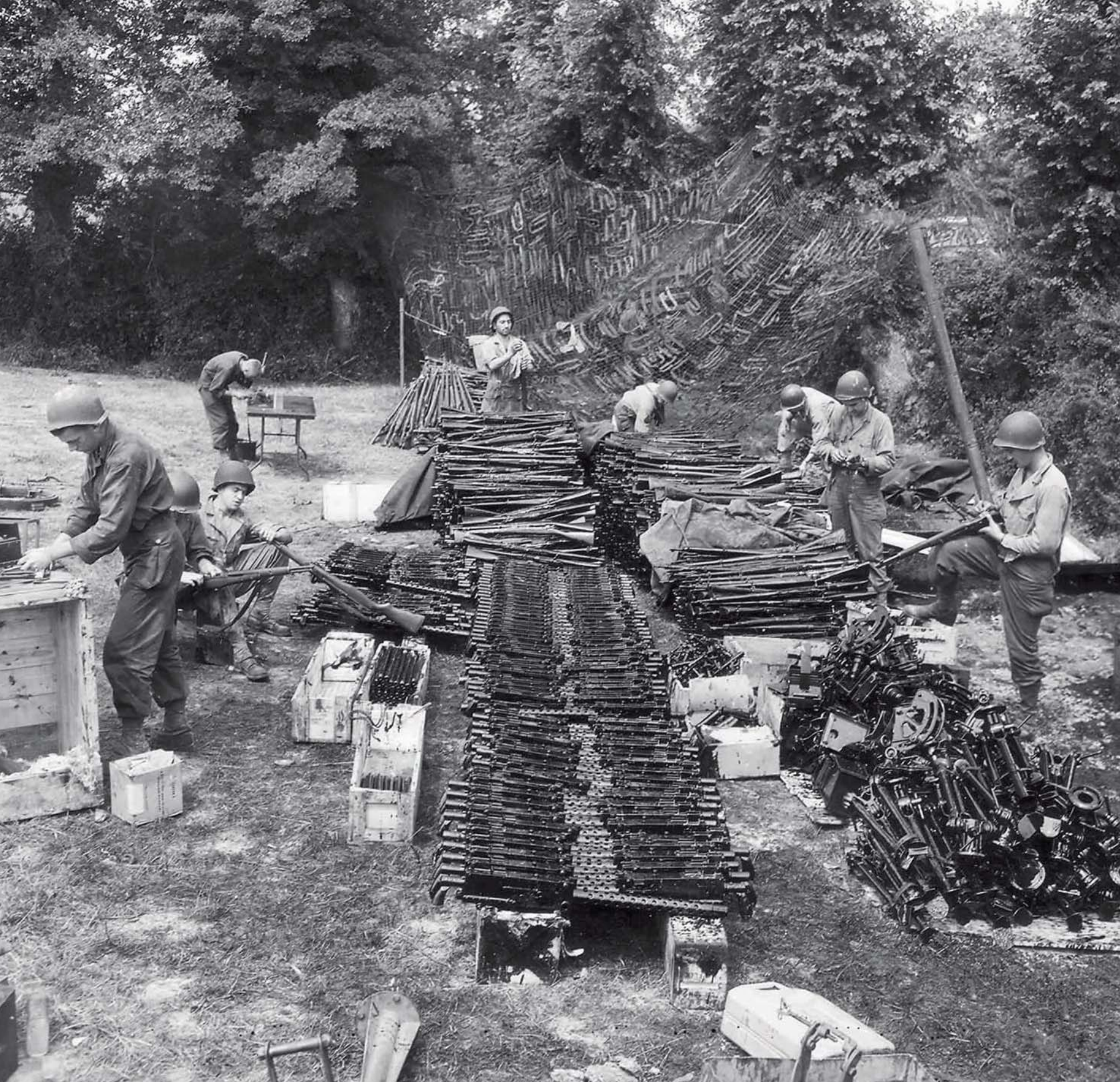
This photograph shows an Ordnance Maintenance and Repair Company at work in a hedgerow-enclosed Norman field on July 18, 1944. One of the U.S. Army's most important types of supporting units, these companies kept the guns running through the intense demands of combat. Among the more striking features of this image are the 116 M1919A4 Machine Guns lined up for servicing and the virtual mountains of M1903 Rifles piled up in front of the camouflage net in the background. Crates of spare M1919A4 barrels and traverse/elevation mechanisms sit close at hand, and, to the right, piles of M2 and M1917A1 Tripods await servicing. The two seated soldiers on the left are cleaning M1 Garand rifles, and the man to the right with his leg up on a crate is doing the same. National Archives and Records Administration/U.S. Army Signal Corps 111-SC-191744
