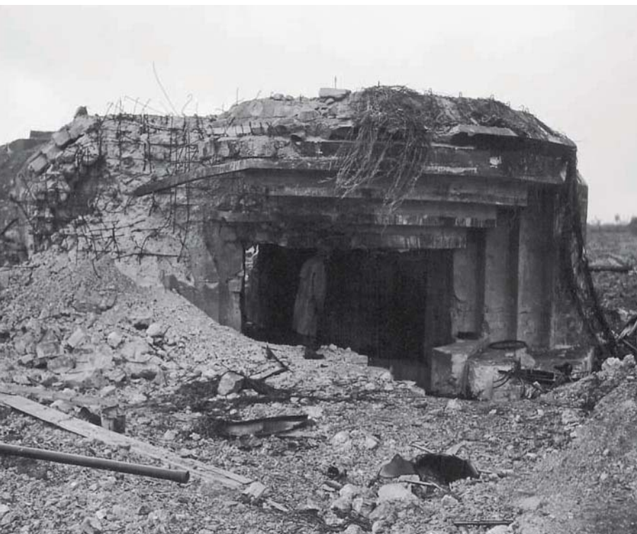
ABOVE LEFT: The battery command and fire control/observation post (a Type R636a bunker) at Stützpunkt Pointe du Hoc (WN75) after the battle. A textured facade has been built around the structure in an effort to camouflage it. National Archives and Records Administration 111-SC-275839 ABOVE RIGHT: One of the Type H679 casemates under construction at Stützpunkt Pointe du Hoc (WN75) when the Rangers landed on D-Day. National Archives and Records Administration 111-SC-275822 BELOW LEFT: Both of the Type H679 casemates at Stützpunkt Pointe du Hoc (WN75) suffered heavy damage during the fighting on D-Day and the days that immediately followed. National Archives and Records Administration BELOW RIGHT: One of the two Type L409A bunkers at Stützpunkt Pointe du Hoc (WN75). This position at one time mounted a 2cm Flugabwehrkanone 30 anti-aircraft gun, but the weapon was removed because of the damage to the concrete. National Archives and Records Administration 111-SC-275825
