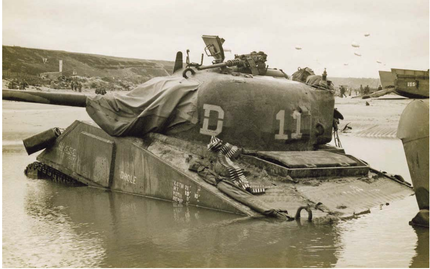
Not every vehicle made a perfect beach landing after D-Day. Here, a split-hatch M4 Sherman medium tank with appliqué armor nicknamed “DHOLE” (D 11) from D Company, 66th Armored Regiment, 2nd Armored Division sits swamped on Omaha Beach on June 10. The tank has the engine exhaust funnel from a deep-water fording kit in place, but there is no air intake funnel. Note the M2HB .50-caliber Machine Gun that has been dismounted and laid on top of the turret as well as the belt of .50-caliber cartridges sitting on top of the vehicle’s engine deck.
