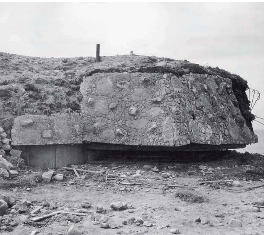
ABOVE LEFT: The battery command and fire control/observation post (a Type R636a bunker) at Stützpunkt Pointe du Hoc (WN75) after the battle. A textured facade has been built around the structure in an effort to camouflage it. National Archives and Records Administration 111-SC-275839 ABOVE RIGHT: One of the Type H679 casemates under construction at Stützpunkt Pointe du Hoc (WN75) when the Rangers landed on D-Day. National Archives and Records Administration 111-SC-275822 BELOW LEFT: Both of the Type H679 casemates at Stützpunkt Pointe du Hoc (WN75) suffered heavy damage during the fighting on D-Day and the days that immediately followed. National Archives and Records Administration BELOW RIGHT: One of the two Type L409A bunkers at Stützpunkt Pointe du Hoc (WN75). This position at one time mounted a 2cm Flugabwehrkanone 30 anti-aircraft gun, but the weapon was removed because of the damage to the concrete. National Archives and Records Administration 111-SC-275825
