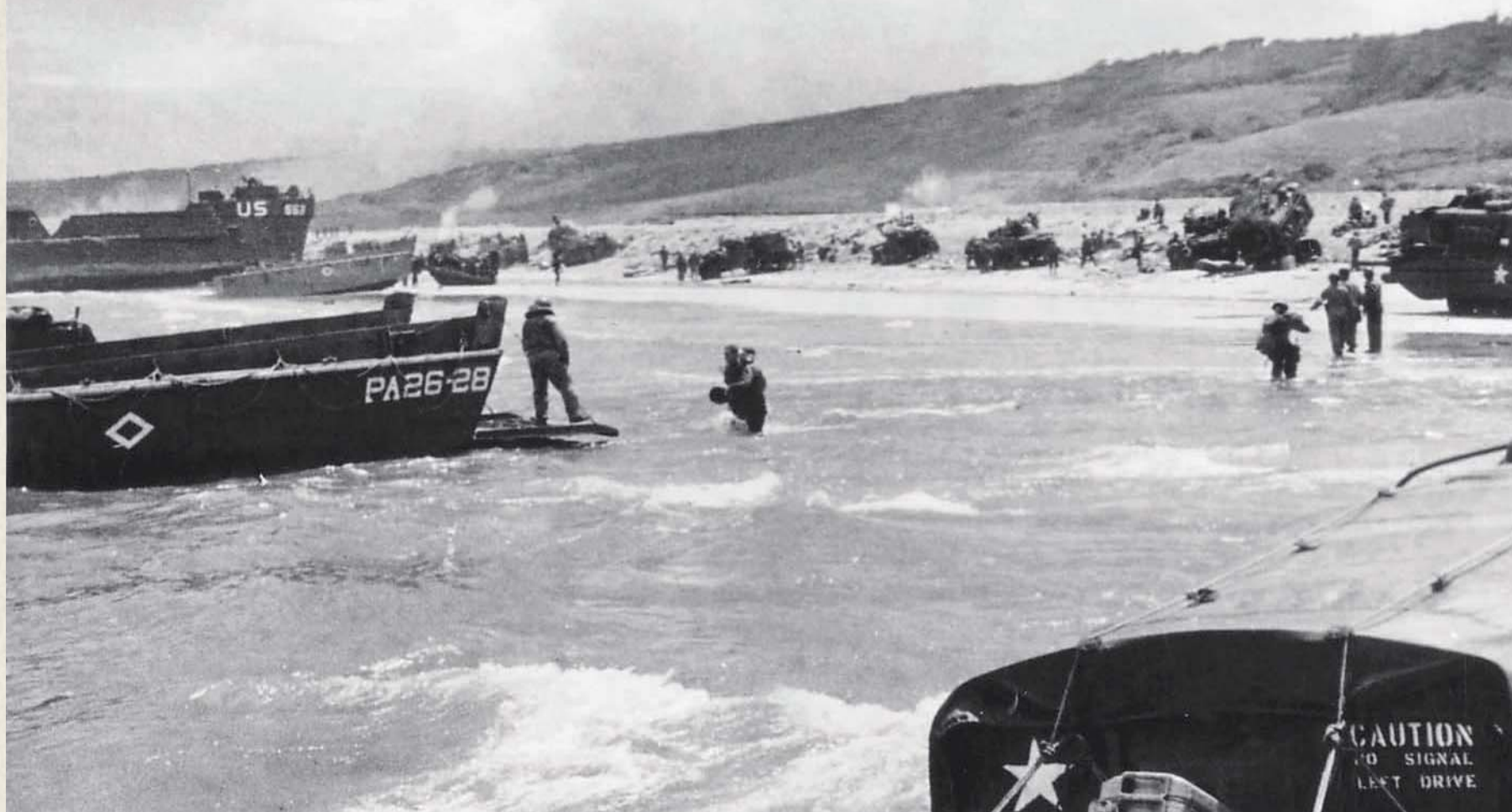
ABOVE: High tide on Omaha Beach is seen here near Exit E-3 shortly before noon on D-Day. The LCVP at left center is from the Arthur Middleton -class attack transport USS Samuel Chase (APA-26), and the larger landing craft above it is LCI(L)-553, which delivered Company H, 115th Infantry Regiment, 29th Division to the beach before being damaged by enemy gunfire. Note the "Caution No Signal Left Drive" sign on the vehicle at the lower right and the DUKW on the beach at the far right. National Archives and Records Administration/US Army Signal Corps 111-SC-189899 BELOW: Another view showing low tide on Omaha Beach after the start of the invasion, looking east toward the Easy Red, Fox Green, and Fox Red sectors. LCVPs, LCTs, DUKWs, and about twenty VLA barrage balloons can be seen here.
