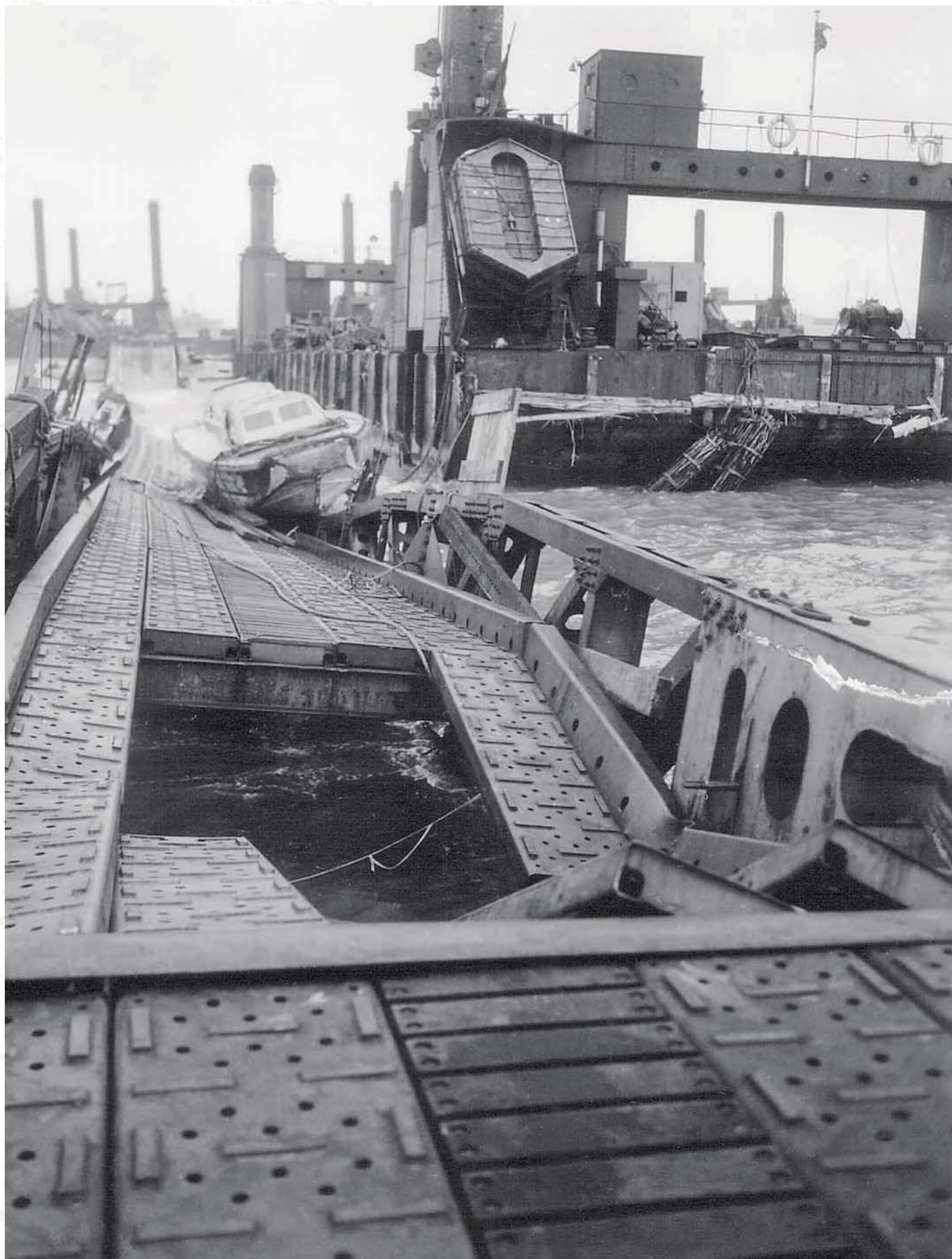
The storm that struck the Baie de la Seine starting on June 19 wreaked havoc on Mulberry Harbor A at Omaha Beach. Here, a Higgins LCS has been pushed up onto one of the whale floating piers, which has been buckled and bent by the pounding surf. Three damaged Löbnitz pierheads can be seen in the background. National Archives and Records Administration/U.S. Army Signal Corps
