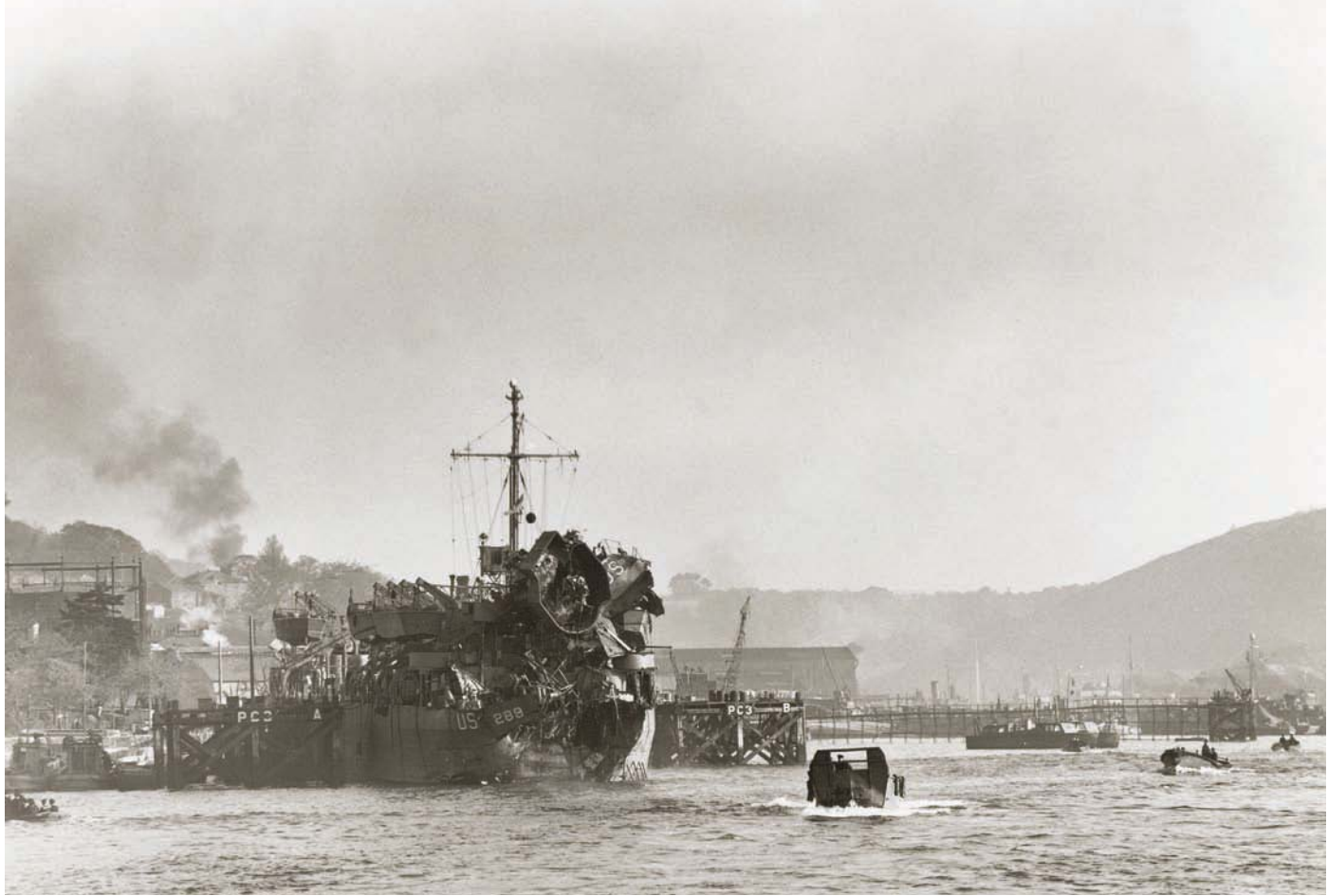
ABOVE: LST-289 is seen here in port at Dartmouth in Devon after being severely damaged by a German E-boat torpedo attack off of Slapton Sands on April 28, 1944, during Exercise Tiger, a rehearsal for the Normandy invasion. BELOW: Close-up of the area of LST-289 showing the heavy damage she sustained during the E-boat attack in Lyme Bay. Thirteen men died in the upturned 40mm gun tub located on the ship's stern.
