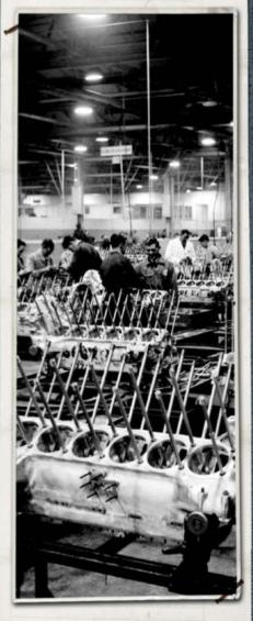
**ABOVE:** The Merlin engine under construction. Here the crank case assembly bay can be seen, with cylinder studs in the process of being fitted.
