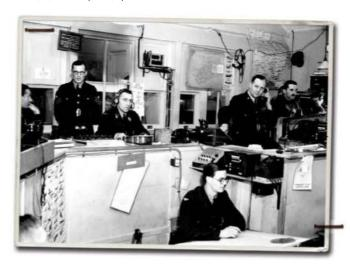
**BELOW:** The Sector "G" Operations Room at Duxford in September 1940. The fighter squadron callsigns can be seen on the wall behind the operator, third from left. The controller is fifth from the left, and on the far right, behind the army liaison officer, are the R/T (Radio Telephone) operators in direct touch with the aircraft.
