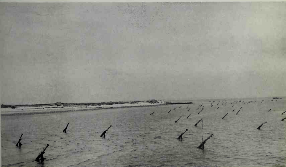
Visible at low tide, slanted poles designed to rip the bottoms from landing craft protected the beaches near Grandcamp-les-Bains. ( Signal Corps, U.S. National Archives )
