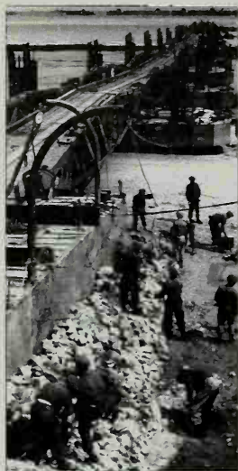
Troops build a caliper wall and bridge to connect with a distant pier
