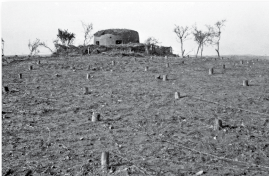
The eastern and western ends of the Cherbourg Landfront were anchored by heavily fortified strongpoints. This is the 40P8 armored cupola of a buried R644 bunker armed with two MG.34 machine guns and a 47mm anti-tank gun. This bunker covered the anti-tank ditch of defense nest W486 in Panzerwerk Westeck near Gréville. This bunker was protected to the higher "A" standard with walls 3.5m thick (11.5ft), making them resistant to almost any type of artillery. This photo was taken in February 1944 and shows the bunker with its full array of barbed wire obstacles in front. (Library of Congress)
